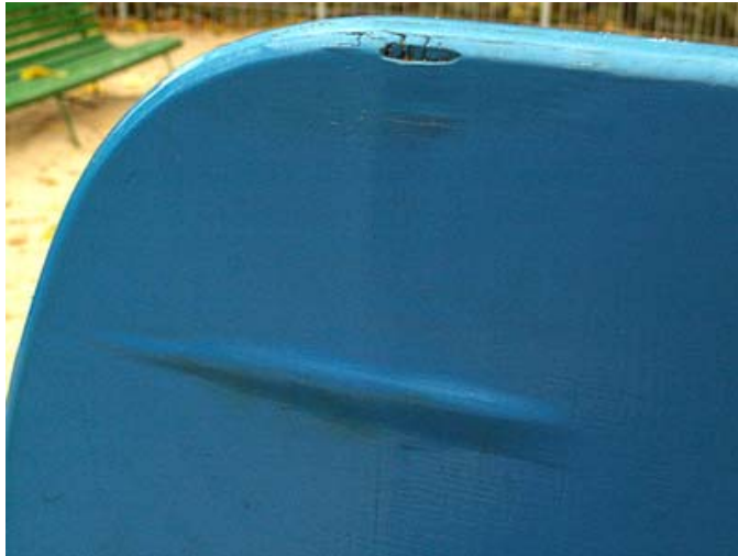
Example of plywood where bad protection of the border caused internal delaminating.
