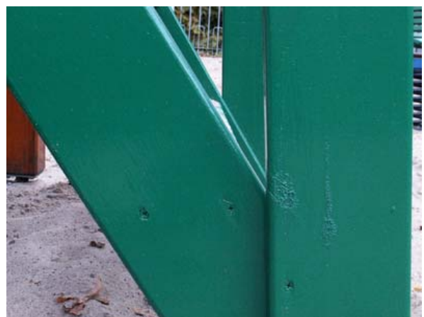
Typical places of jamming: at joints of two diagonal rungs (the picture was taken during examination of possibility of head jam) and at the end of steps.
